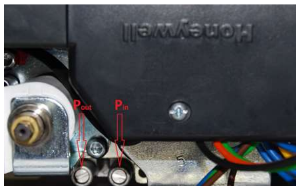
Photo 3 - Nozzles measuring gas pressure
